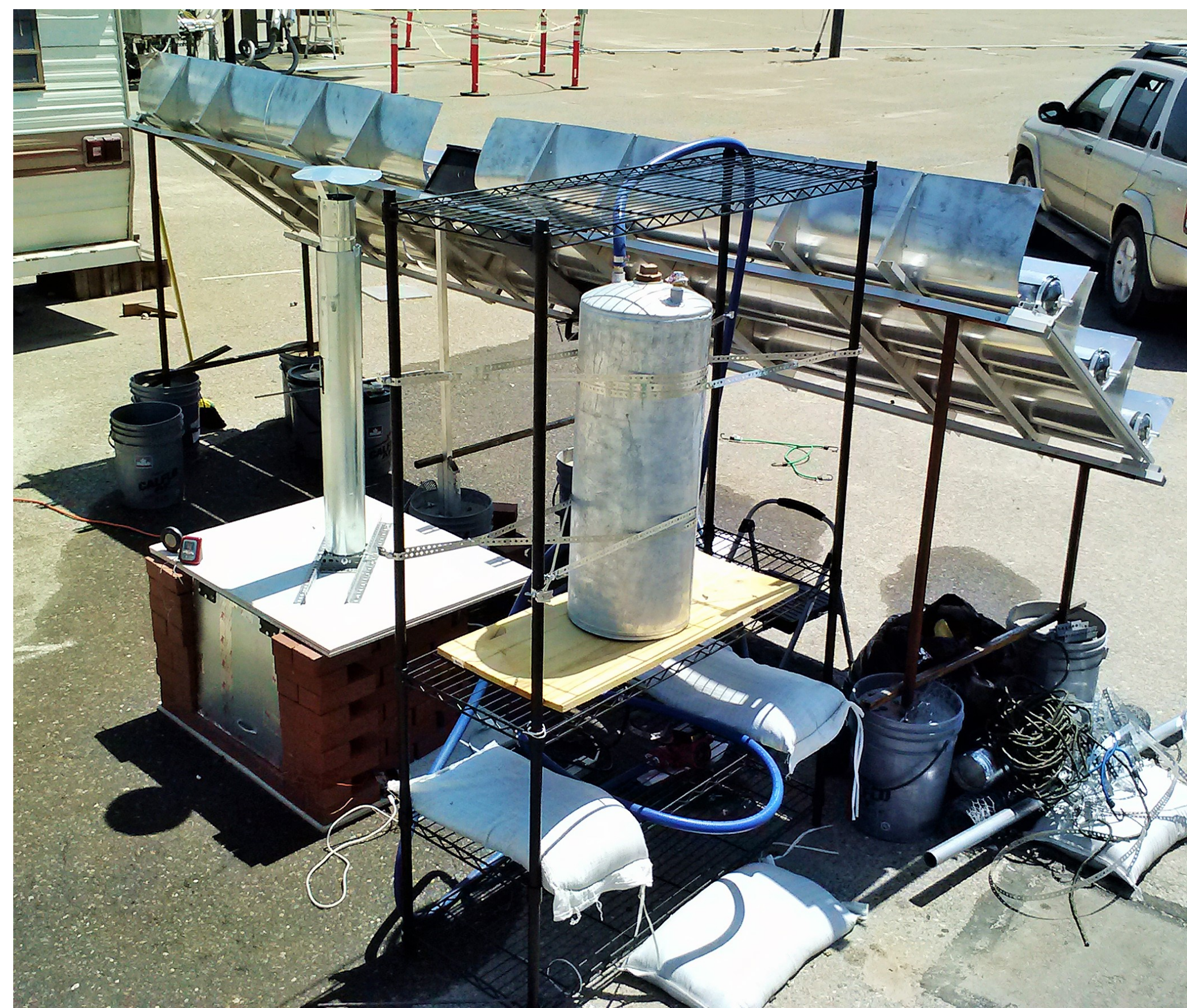
Figure 2. Picture of Solar Waste Solution System at UC Merced Castle Facility
